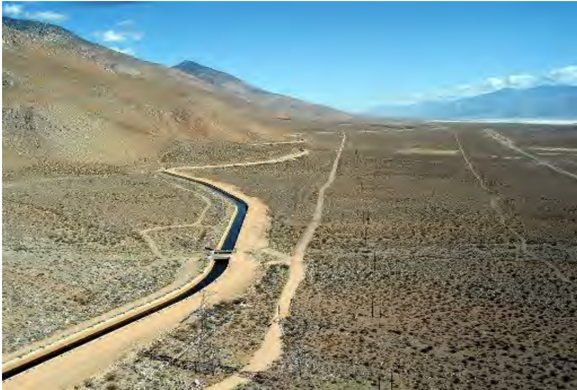
Figure 35. Los Angeles Aqueduct – it runs south through Owens Valley desert on its way to distant L.A.
